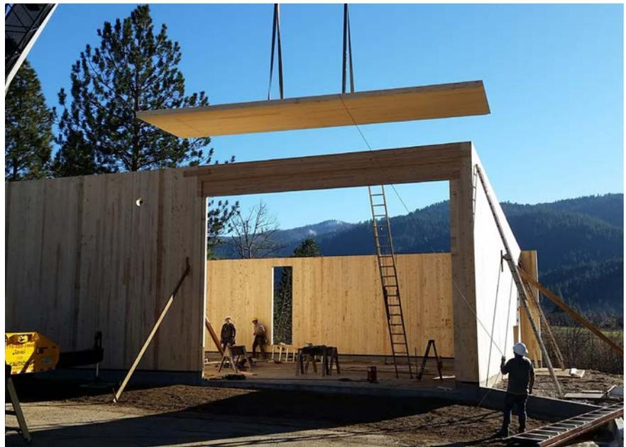
*CLT wall and roof panel being hoisted into place at California's first all CLT building in Quincy, CA*
